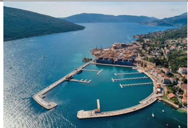
Figure 13. Seaport structures – Porto Novi https://www.total-montenegro-news.com/business/2956-portonovi-hn
