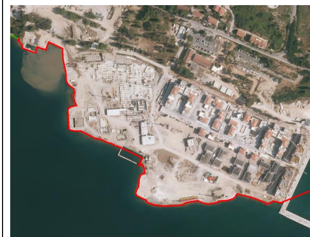
Figure 21: Construction works near the coastline – Kumbor- Porto Novi
