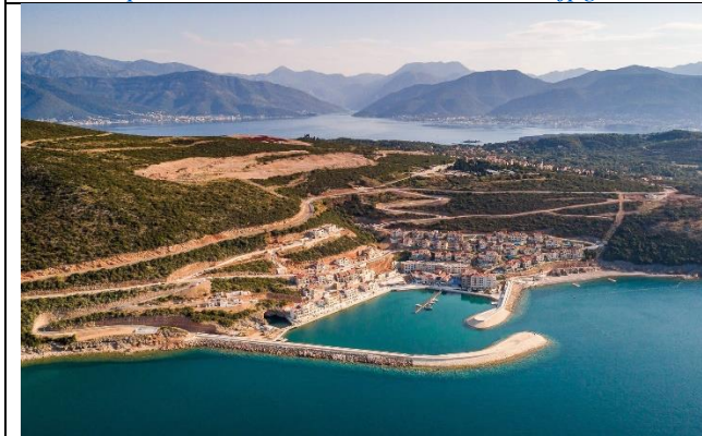
Figure 12. Turističko naselje Lištica Bay – breakwaters - seaport structures https://www.build-review.com/lustica-bay-montenegro-over-100-percent-increase-in-prices-in-seven-years-and-highly-competitive-rental-yield-among-highest-in-europe/
